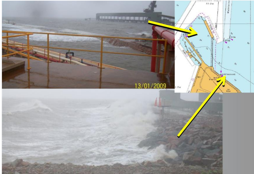
Figure 2. Wave conditions behind berth 11 in front of the breakwater (top) and those in front of the reclamation revetment (bottom)
